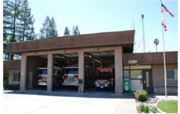
STATION 41 1280 Moraga Way, Moraga
