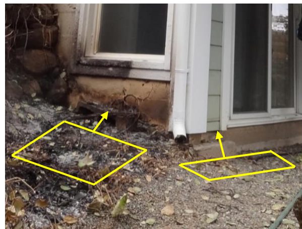
Figure 5a-b. Example of vegetation in small amounts located in Zone 0 creating a pathway for fire spread: (a) Wood mulch provided a pathway for fire to get close to the building and ignite a hot tub during the Glass Fire (2020) in Napa and Sonoma Counties, California; (b) Ground-level plants during the Glass Fire (2020).
