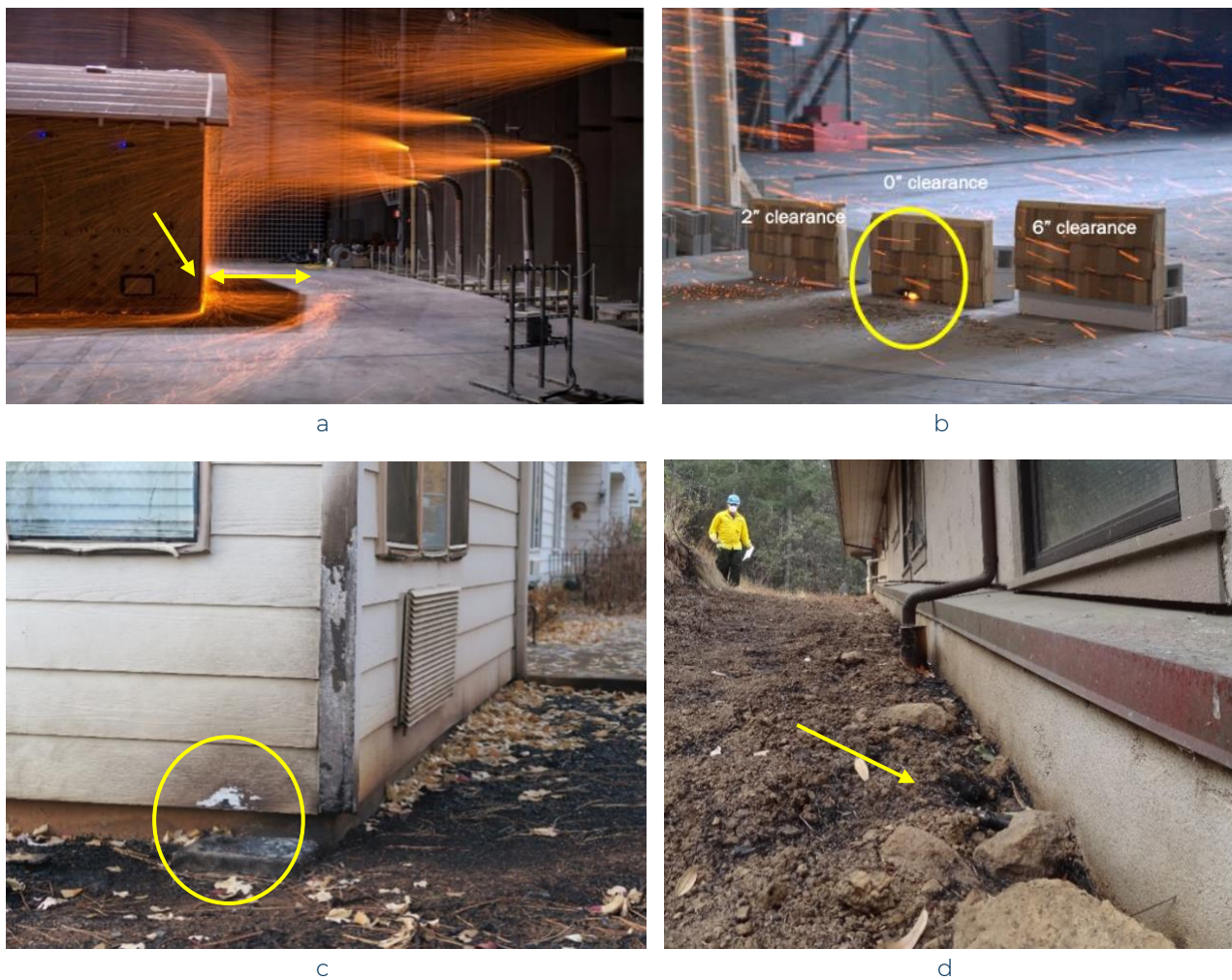
Figure 4. Ember accumulation at the base of the wall causing ignition (a and b) at the IBHS Research Center, (c) in the post-Camp Fire (2018) investigation in Butte County, California, and (d) at the base of a wall in the Glass Fire (2020) in Napa and Sonoma Counties, California, which did not have the opportunity to grow because of a noncombustible vertical clearance.
