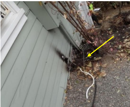
Figure 5a-b. Example of vegetation in small amounts located in Zone 0 creating a pathway for fire spread: (a) Wood mulch provided a pathway for fire to get close to the building and ignite a hot tub during the Glass Fire (2020) in Napa and Sonoma Counties, California; (b) Ground-level plants during the Glass Fire (2020).
